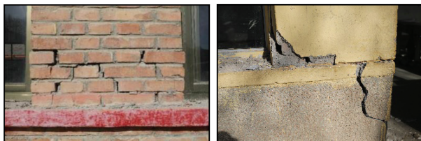
(a) 窗间墙(柳沟乡, VIII度) (b) 门窗洞口间墙体(柳沟乡, VII度)
