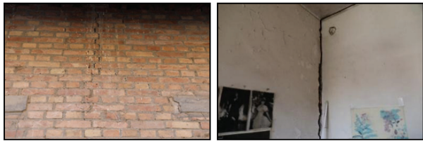
(a) 竖向沿齿裂缝(柳沟乡, VIII度) (b) 墙体外闪(柳沟乡, VIII度)
